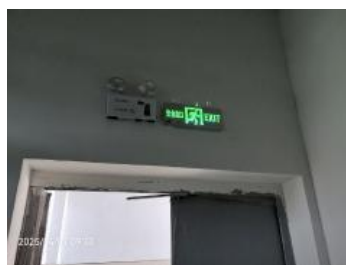
safety exit sign and emergency light.jpg
