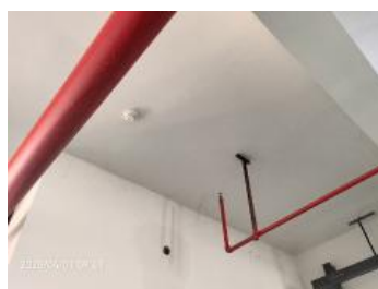
fire sprinkler and smoke alarm.jpg
